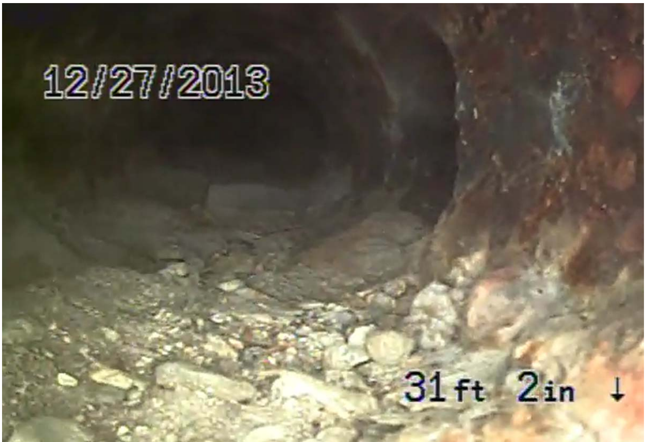
Screen shot 28: four-inch cast iron pipe drain line 8 beneath Building 3, note depression in pipe sediment suggesting a potential hole in the pipe bottom
