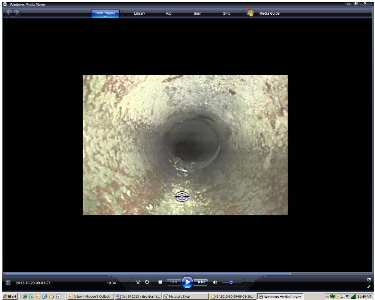
Screen shot 8: clear section of four-inch clay pipe drain line 4
