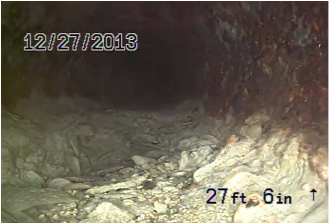
Screen shot 28: four-inch cast iron pipe drain line 8 beneath Building 3, note depression in pipe sediment suggesting a potential hole in the pipe bottom
