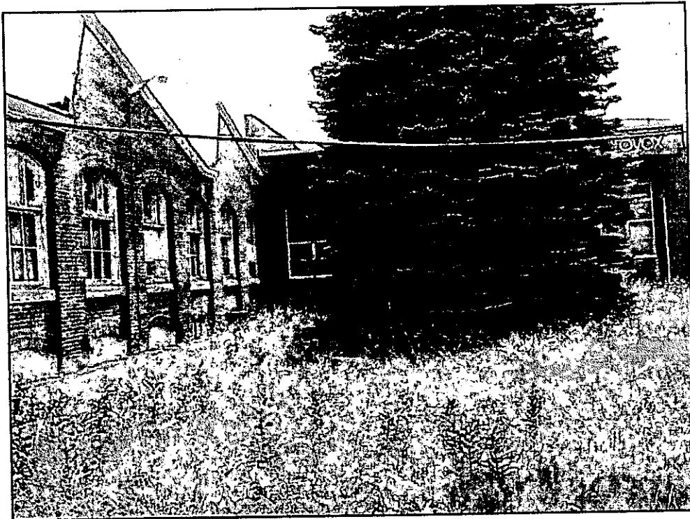
SCENE: View of the northwest corner of the Aerovox building. Photograph taken facing south.
