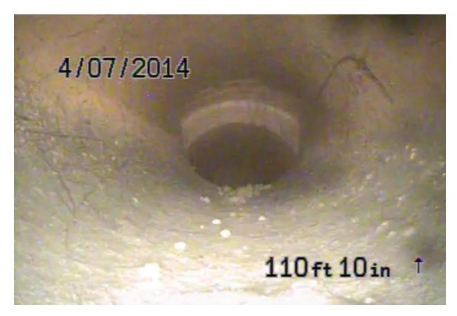
Screen shot 9: four-inch clay drain line 9 at Building 3 with significantly off-set joint, approximately 110 feet from former sump
