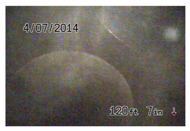
Screen shot 14: ten-inch clay drain line 10 at Building 5 with potential roof drain connection at upper right, approximately 120 feet from manhole
