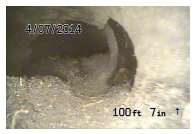
Screen shot 8: four-inch clay drain line 9 at Building 3 with potential break on right, approximately 100 feet from former sump
