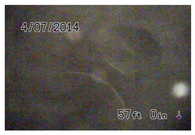
Screen shot 12: ten-inch clay drain line 10 at Building 5 with potential roof drain connection at upper right, approximately 57 feet from manhole
