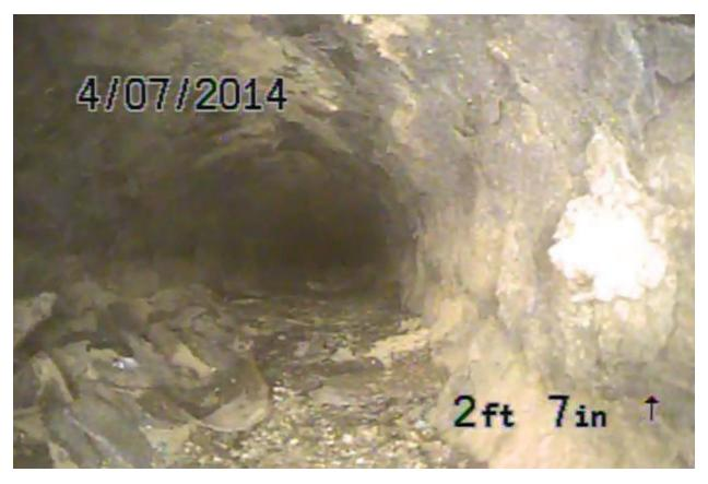
Screen shot 1: four-inch cast iron drain line 7 at Building 3 with wall deposits and sediment before cleaning
