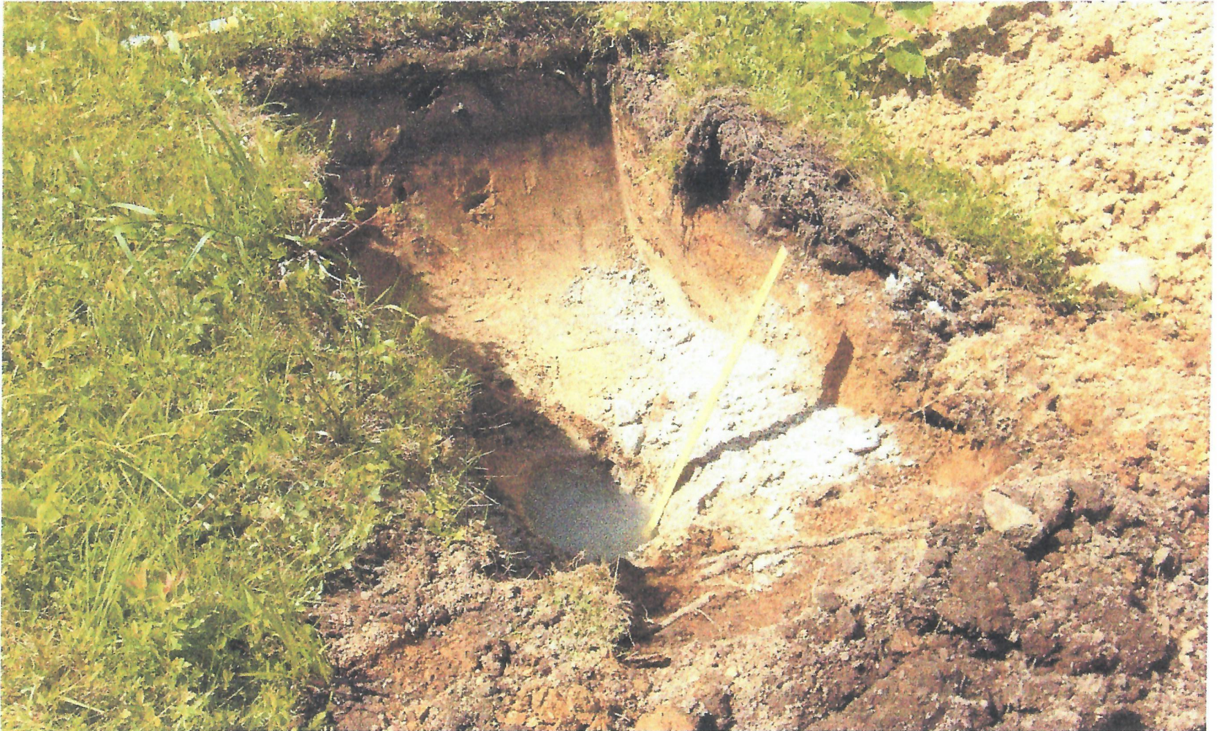
Perc Test #1 Shutesbury Library 60 Leverett Road Shutesbury MA 06.29.2010
