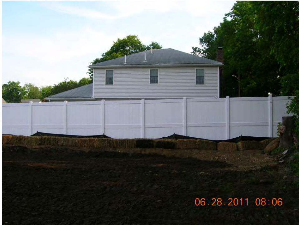
SCENE: View of the new fence at 53 Hoffman Avenue. Photograph taken facing north.
