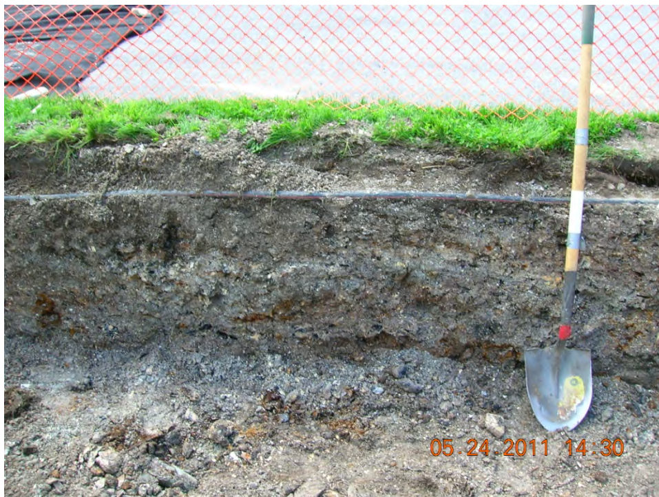
SCENE: View of the ash layer beneath the driveway at 33 Hoffman Avenue. Photograph taken facing west.
