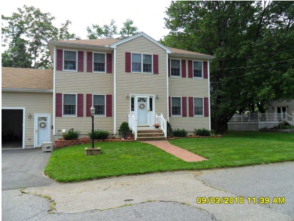
SCENE: View of 33 Hoffman Avenue. Photograph taken facing south.
