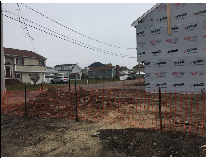
Subject Property, looking north, west side of building exterior
