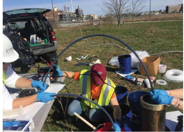
Photo 2: MW-414 – NAPL pumping, 4/17/17.
