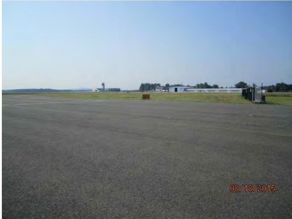
Photo 1: Former FTA-01 (IRP Site 1) Looking South
