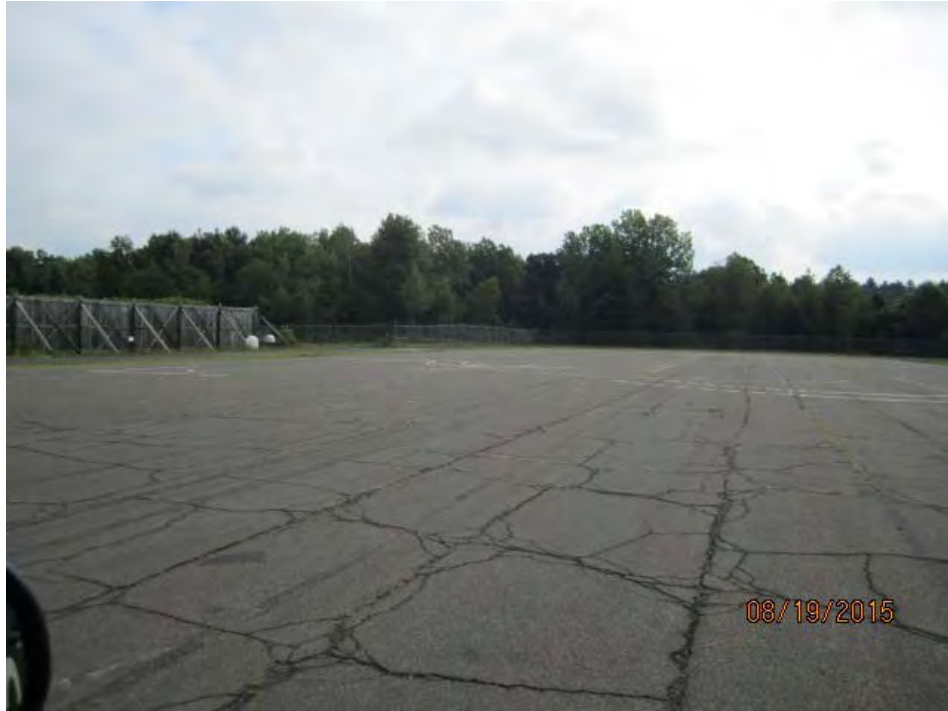
Photo 5: Fire Department Equipment Test Area – East End of Sierra Taxiway
