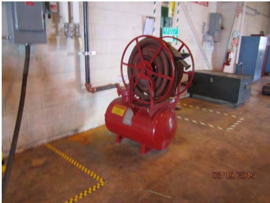
Photo 4: AFFF Deck Gun (four total) - Hangars 27A and 27B
