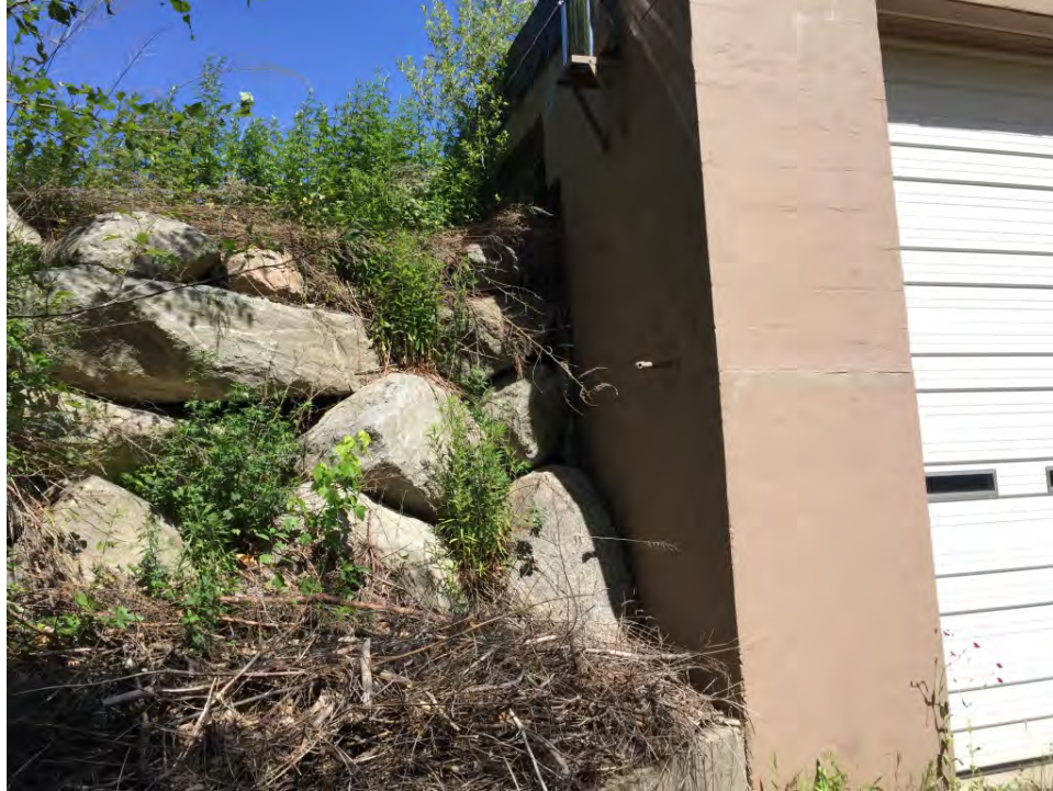
SCENE: View of the large boulders used as fill material observed near the residence. Photograph taken facing northwest.
