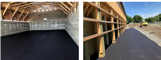
Note: New shed completed in Medford with raised ceiling and new floor.
