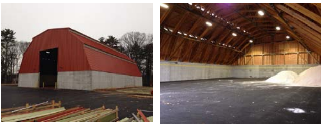
Note: New shed completed in Billerica allows for spreader trucks to be loaded under cover.
