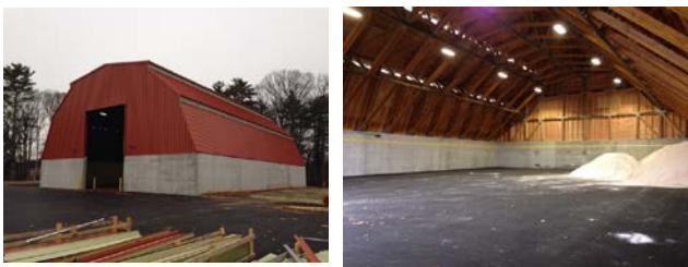
Note: New shed completed in Billerica allows for spreader trucks to be loaded under cover.
