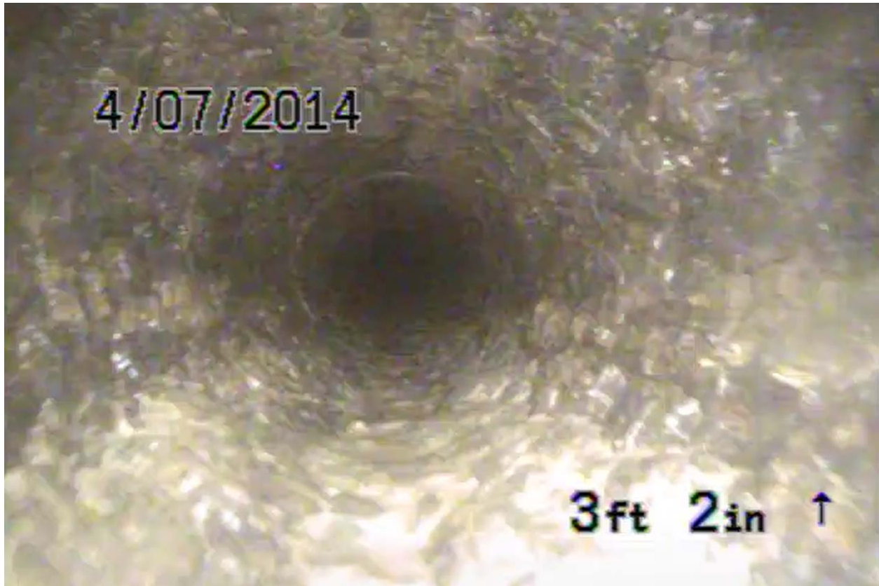
Screen shot 2: four-inch cast iron drain line 7 at Building 3 after cleaning
