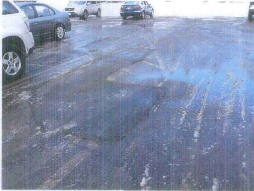
Area 8 Pavement Repair
