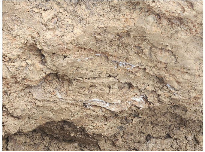
Side wall of excavation showing ACM imbedded in soil.
