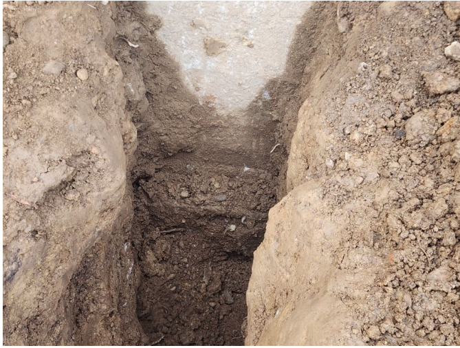
Asbestos containing material (ACM) encountered at approximately 3 feet deep.
