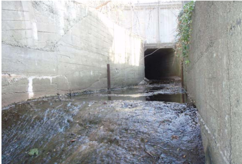
Photo 1. Storm drain daylight location.
