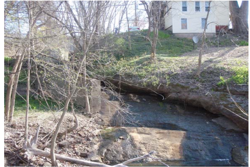
Photo 2. View of outfall and ponding area below.
