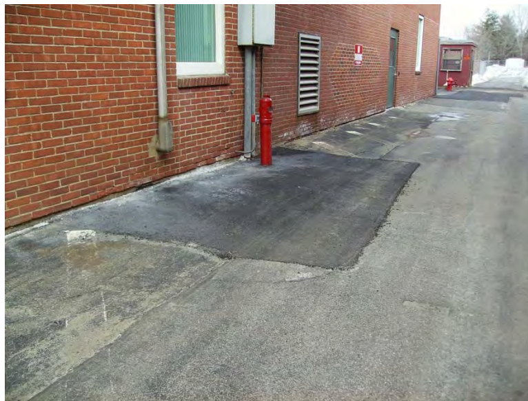
URAM Excavation Area 2
