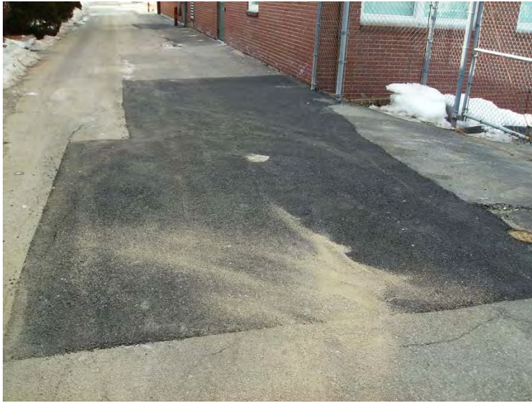
URAM Excavation Area 1
