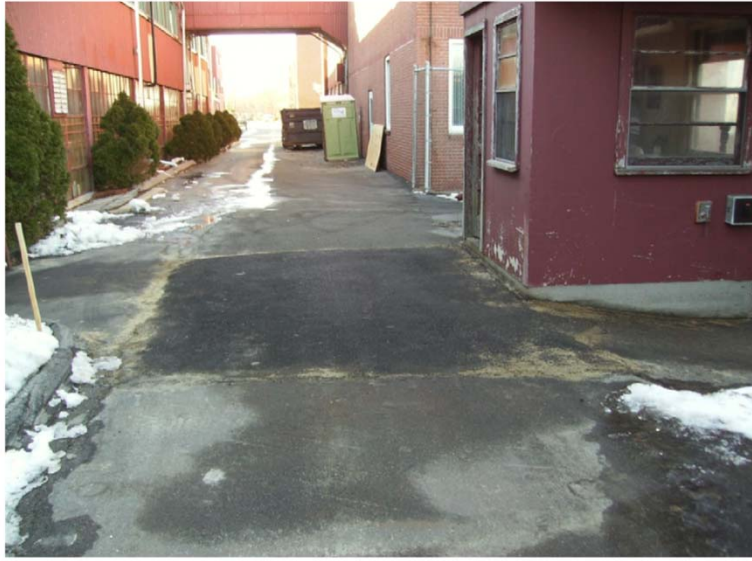
Fire Suppression Leak Area (RTN 3-31257)
