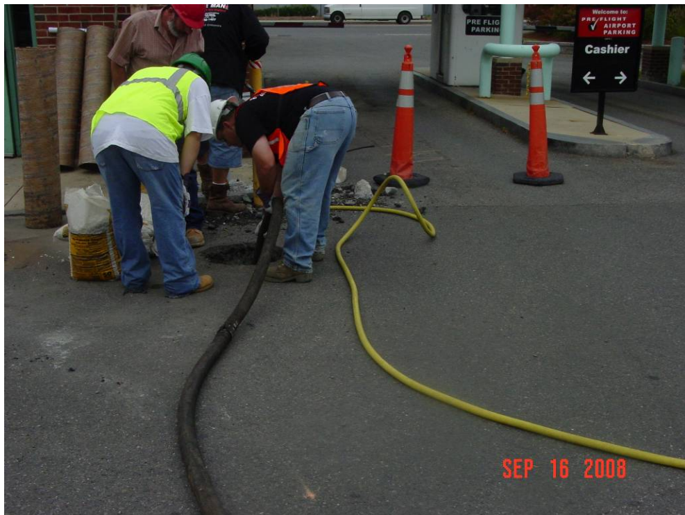
Groundwater being vacuumed out of a Borehole.
