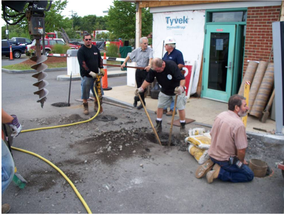
Installation of Sonotube (Office Building to right-looking southwest).
