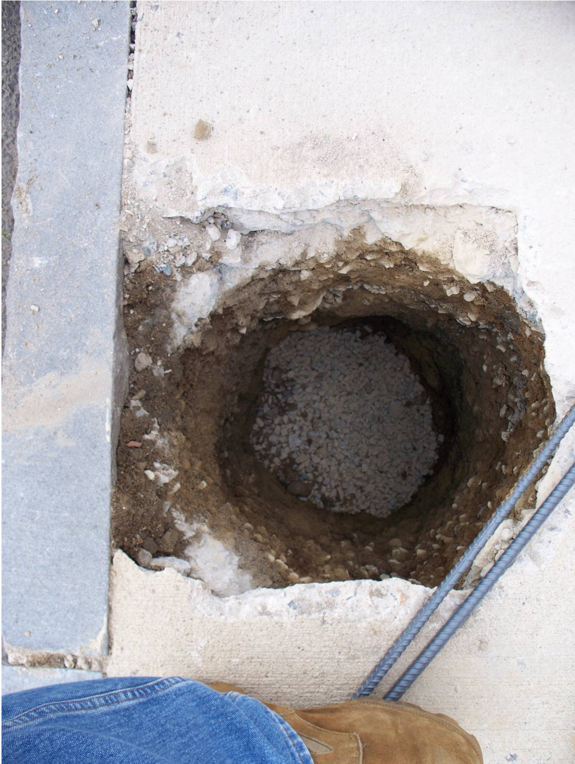
Gravel at base of Borehole preparatory for concrete base for pier.
