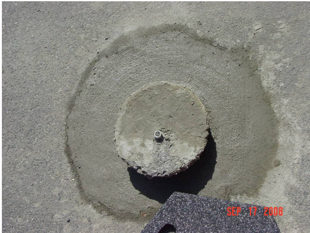
Finished Pier Installation (typical).
