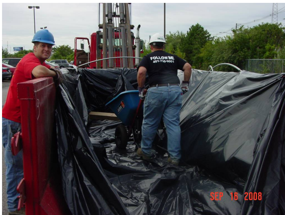
Remediation Waste Soil being placed in Lined, Gasketed Roll-Off
