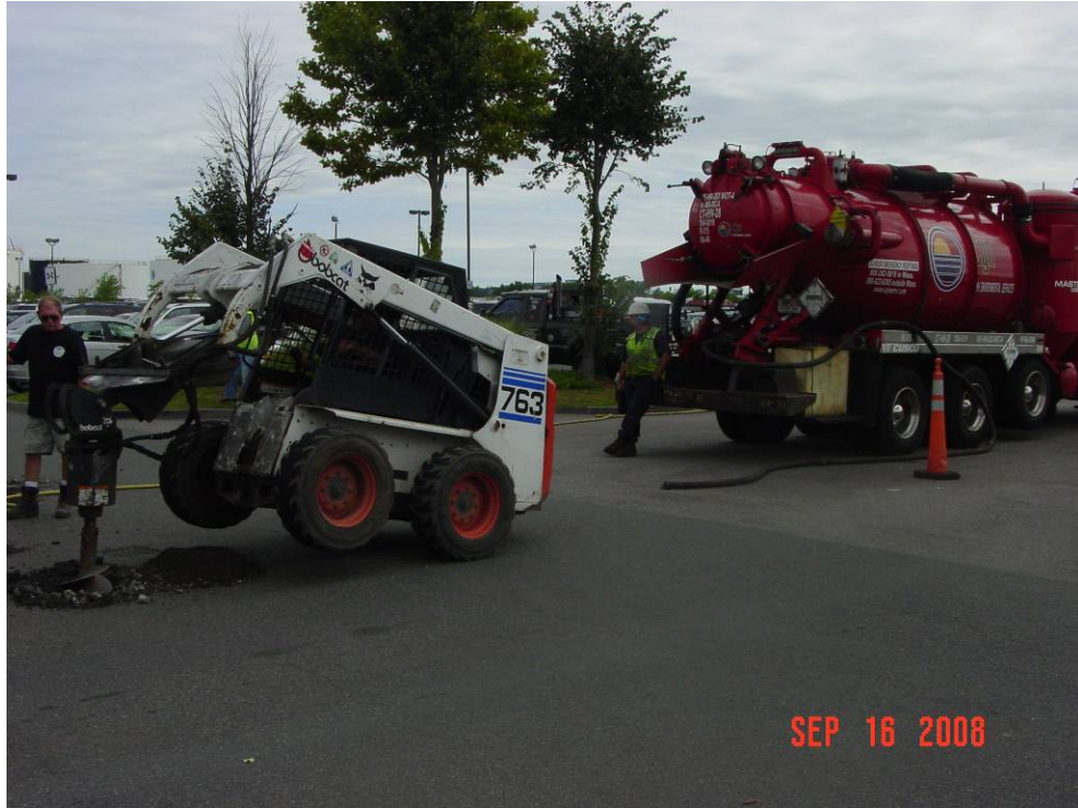
Bobcat® and Vactor 722 Vacuum Truck (looking northeast)
