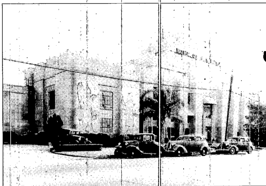
The Assyrian-style administration building shown in this photo from the 1930s is all that remains of the former Uniroyal complex in the City of Commerce, Calif. Trammel Crow, a redevelopment firm that spent $85 million to demolish and refurbish the property, retained the office structure and a 1,700-ft. wall because they were well-known landmarks in the community. The firm leases the multiuse site from the city.
